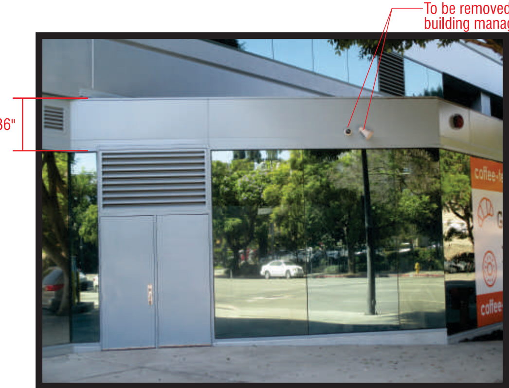
Existing North Elevation- 3rd Street (Close-Up)
