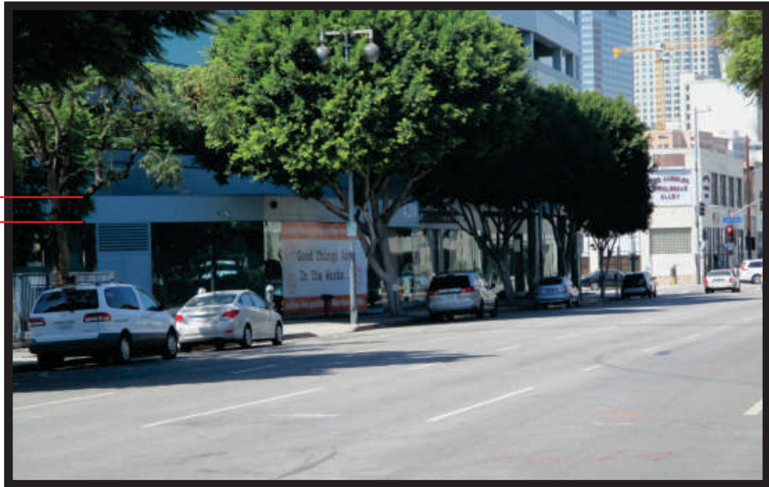
Existing North Elevation - 3rd Street (Overall)
